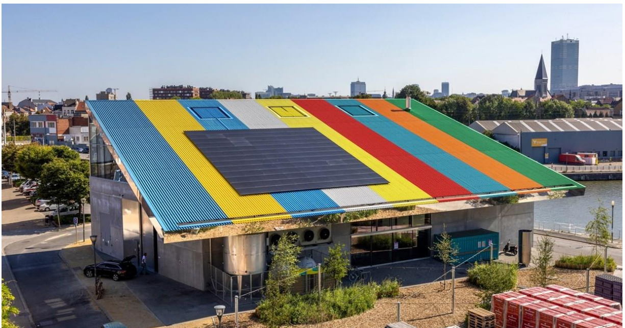
Figuur 17: Brussels Beer Project Port-Sud, Brussel – Office KGVDS
